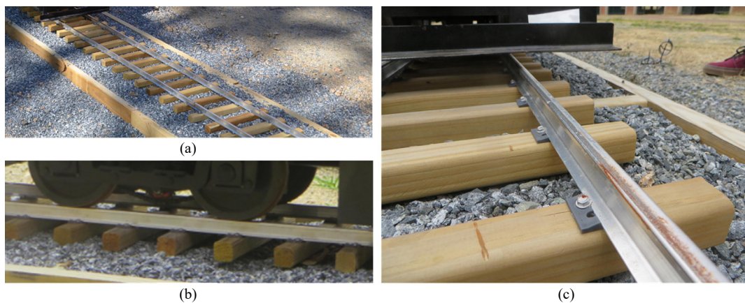
Figure 2. Conventional aluminum railroad track for MPM
