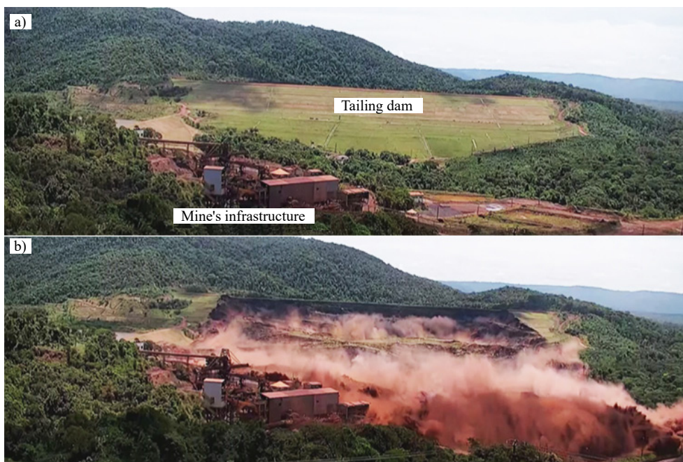
Figure 1. (a) Accident area and (b) mudflow seconds after the mining tailing dams failure [1]
