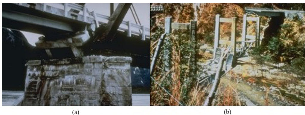
Figure 1. Damaged Bridges: (a) Support damage of the Copper River bridge due to rocking, Alaska 1964 (from USGS Earthquake Hazards Program), and (b) Overturning of three spans of the Agua Caliente Bridge, Guatemala, 1976 (from Public Roads 40(3), pp.101-107, by J.D. Cooper) - reproduced from reference [3]
