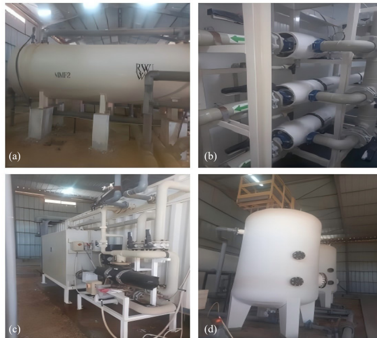
Figure 2. (a) Multi-media filtration units, (b) Cartridge filters, (c) Clean-in-place (CIP) system, (d) Calcite units
