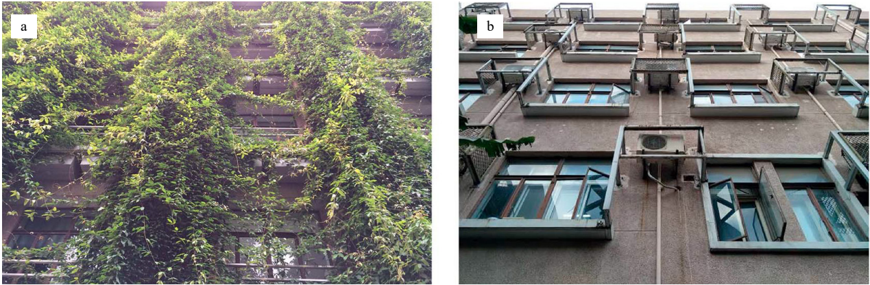
Figure 4. (a) DSGF and (b) original bare facade [22]
