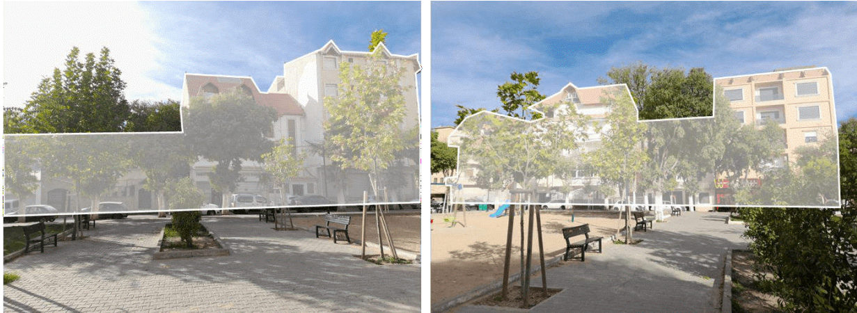
Figure 8. Photographs illustrating the heterogeneity of building types on the east and west facades
