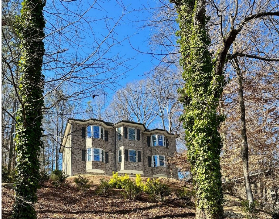
Figure 5. Outside picture of the house
