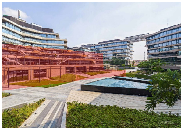
Figure 9. Office outdoor extensions [13]
