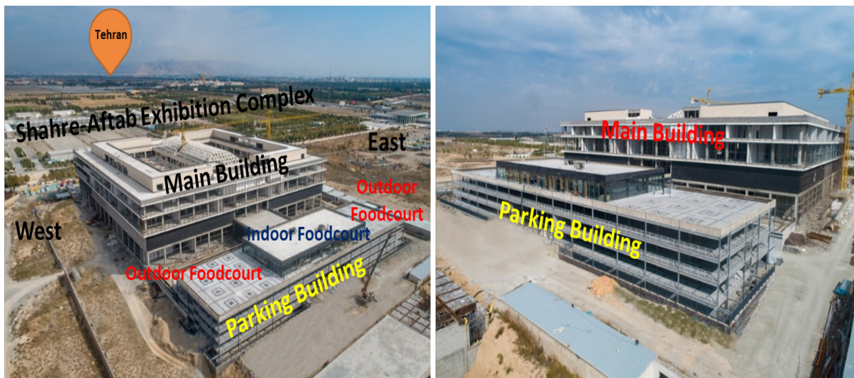
Figure 3. Actual prototype in construction phase
