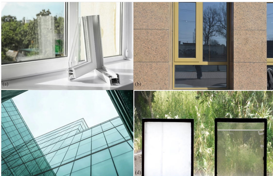
Figure 2. Advanced glazing technologies for mitigating thermal bridges, including a) vacuum glazing, b) vacuum PV glazing, c) low-e coating glazing, and d) PCM glazing in solid (left) and liquid (right) states [64]
